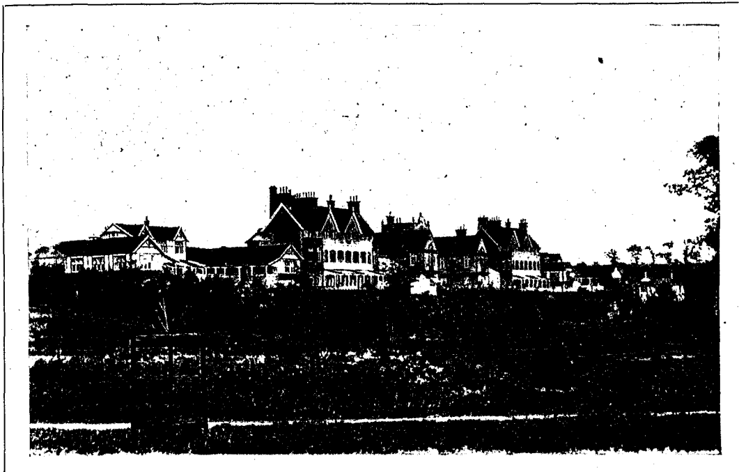
THE ROYAL NATIONAL HOSPITAL FOR CONSUMPTION, IRELAND.
